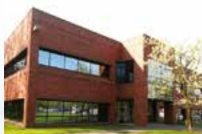
FLIR Systems, Portland
